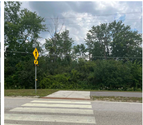
RRFB and marked crossing on Main St
