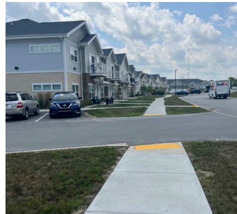
New sidewalk installed in the Rock Pointe Apartments complex
