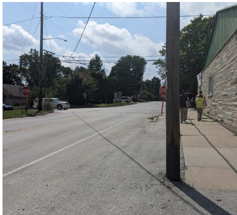
Incomplete sidewalk and pedestrian paved shoulder on Lannon Rd
