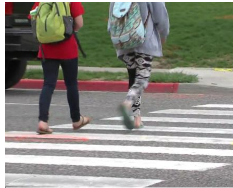
High visibility, ladder-style crosswalk
