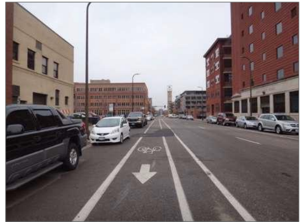
A painted buffer provides extra distance between the bicycle lane and motor vehicle travel lanes on Portland Avenue in Minneapolis.
