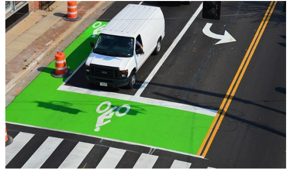
An example of a bicycle box implemented in the City of Wauwatosa, WI
