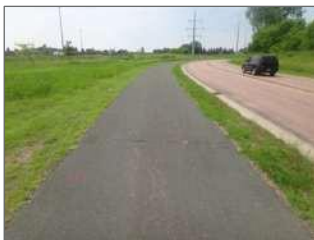
Shared-use path (no lane markings)
