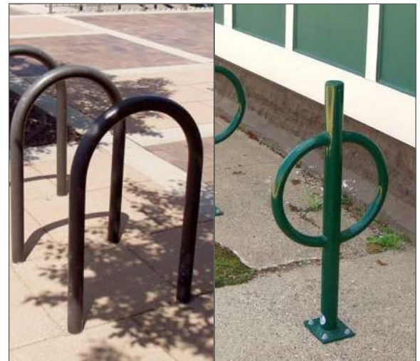
Two of the preferred types of bicycle rack: the "Inverted U" (left) and the "Post and Loop" (right).
