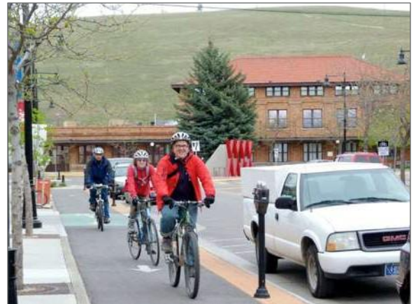
A protected bicycle lane in Missoula, Montana is physically separated from motor vehicle traffic by a curb and parallel parking. Image courtesy of bicycleleague.org.
