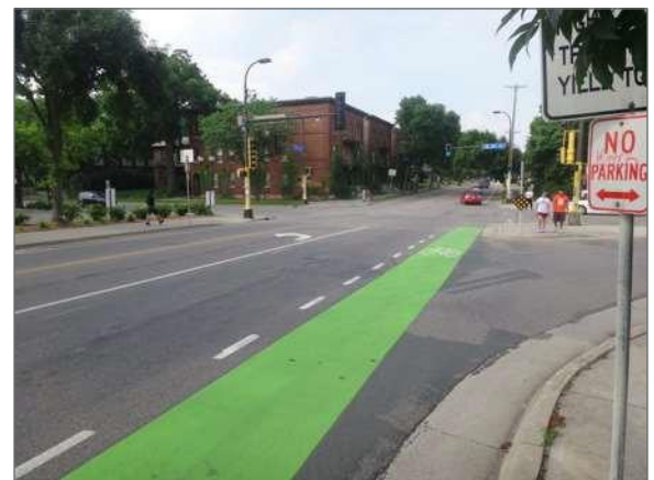
Green painted lanes approaching an intersection in Minneapolis, MN. At this location, motor vehicles travel across the bicycle lane to turn right.
