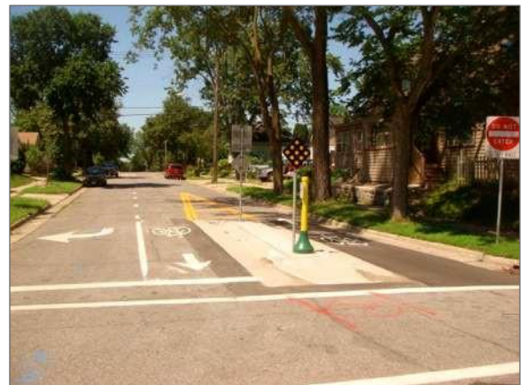
The Riverlake Greenway Bicycle Boulevard in Minneapolis, MN includes traffic diverters to reduce motor vehicle cut-through traffic.
