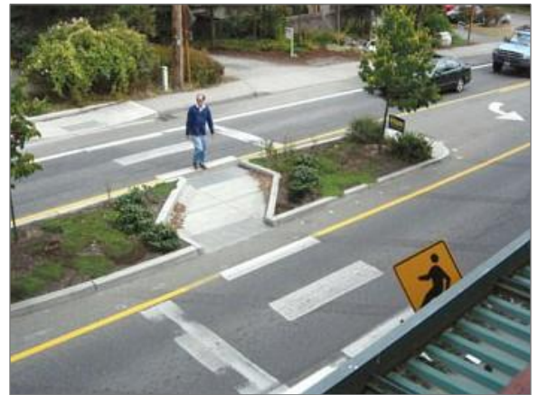
Median crossing island on Bainbridge Island in Washington State. Image courtesy of FHWA.
