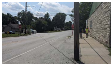
Incomplete sidewalk and pedestrian paved shoulder on Lannon Rd
