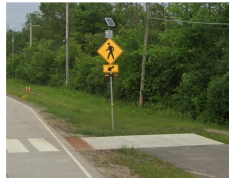
RRFB located at Main St shared use path crossing
