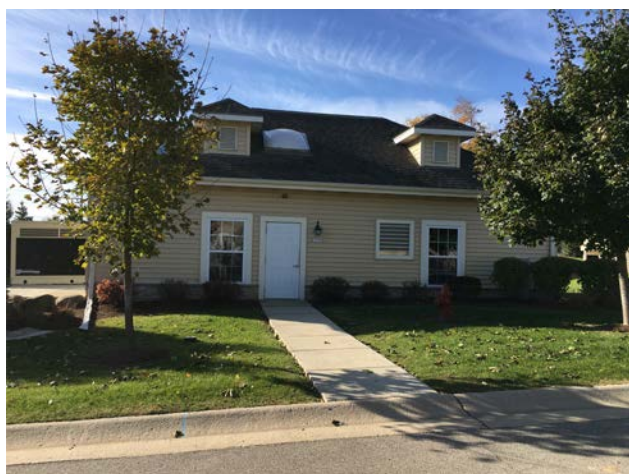
Figure 2.02-1 Well and Booster Facility
