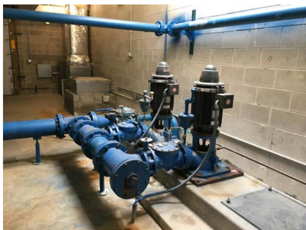
Figure 2.03-1 Booster Pumps
