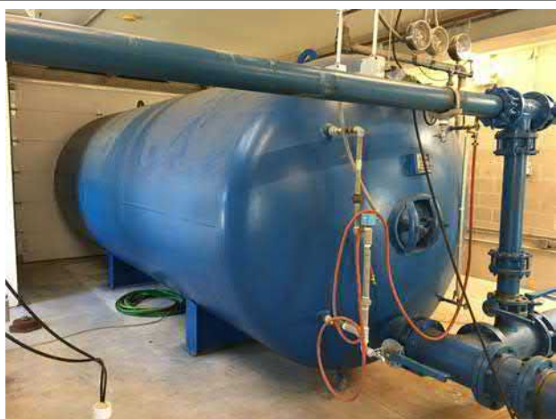
Figure 2.04-1 Pneumatic Pressure Tank
