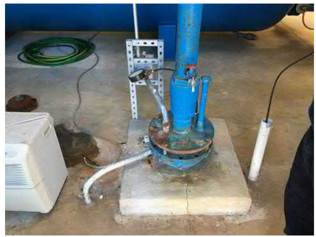
Figure 2.02-2 Well Discharge Piping
